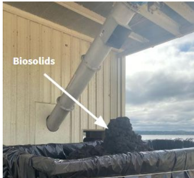
Figure 5. Biosolids produced from CU WWTP awaiting transport to the Anderson landfill
